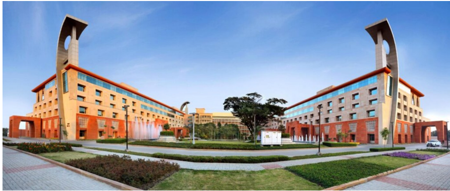
Figure 2: Vallabh Bhawan, Madhya Pradesh
